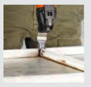
Weathered windows are often restored individually when renovating listed properties. With the E-CUT universal saw blade, you can precisely cut out damaged wing parts and replace them with new wooden parts.
