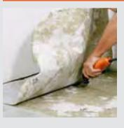
The stopper knife can remove carpet, linoleum or PVC floor coverings, tile adhesive and plaster.
