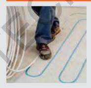
A 1/2 or 3/4 inch plastic water pipe is laid in the individually made cut-out (Ø approx. 25 mm).
